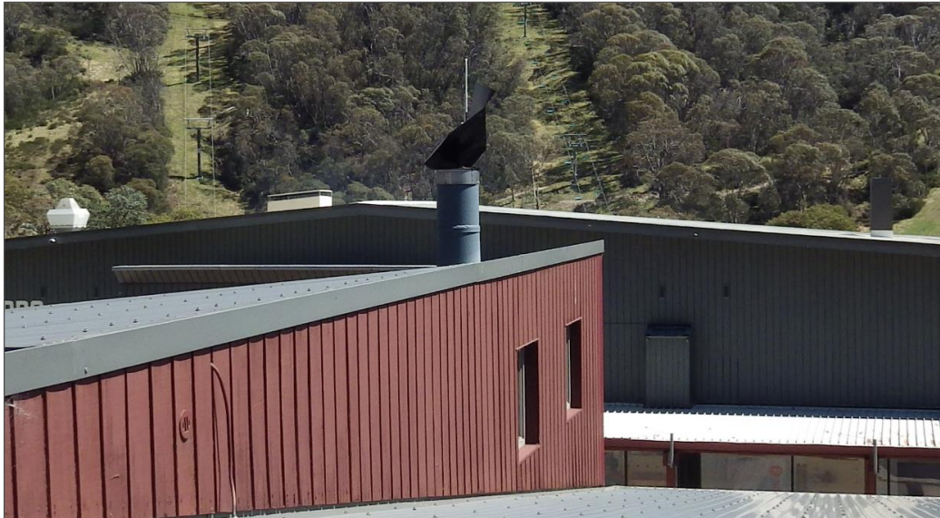
Figure 3 | Former fireplace flue (Source: Department file)
