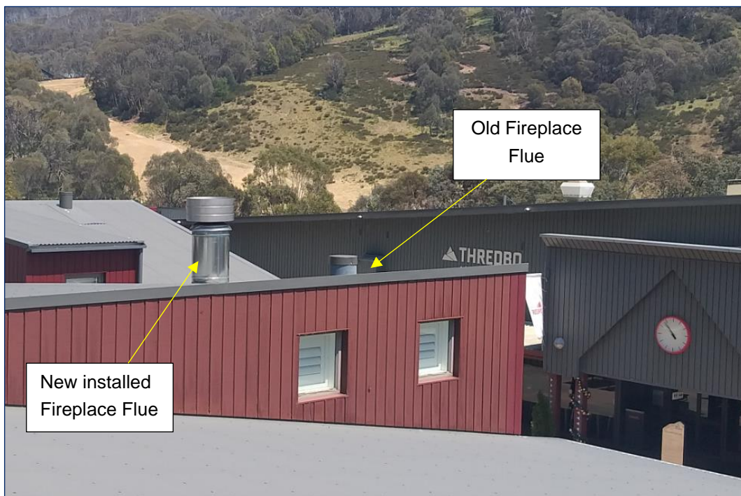
Figure 4 | External works undertaken, installation of new fireplace flue (Source: Department inspection)
