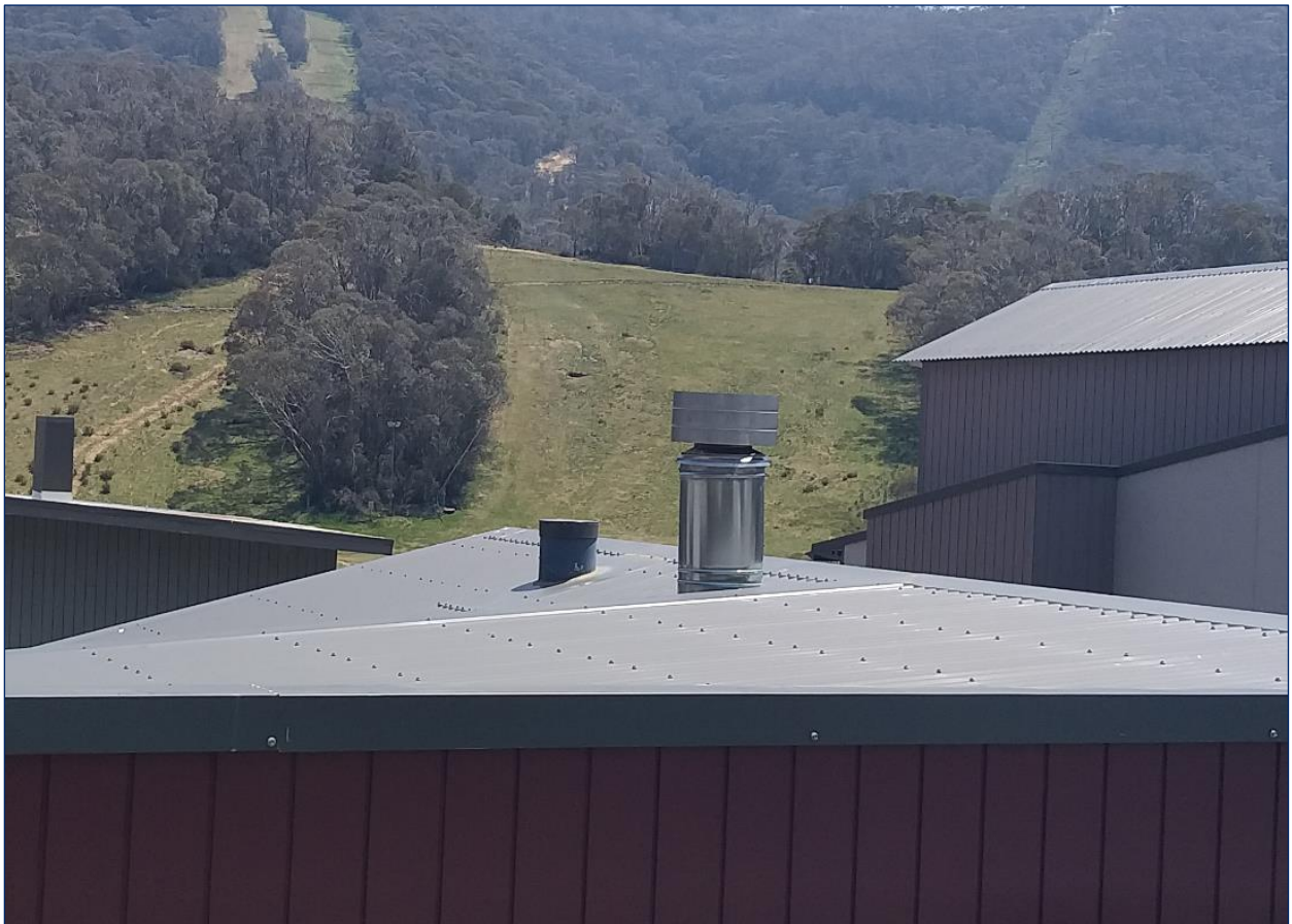
Figure 5 | Existing external fireplace flues subject of application (Source: Department inspection)
